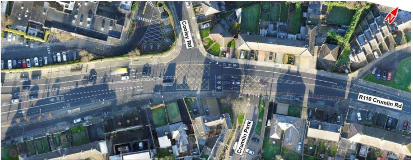
Image 5.25: R110 Crumlin Road / Cooley Road Signalised Junction
