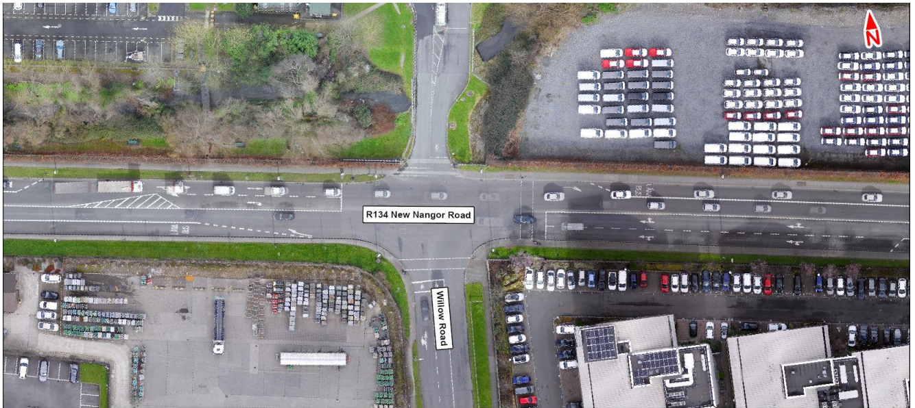
Image 5.44: R134 New Nangor Road / Willow Road Signalised Junction
