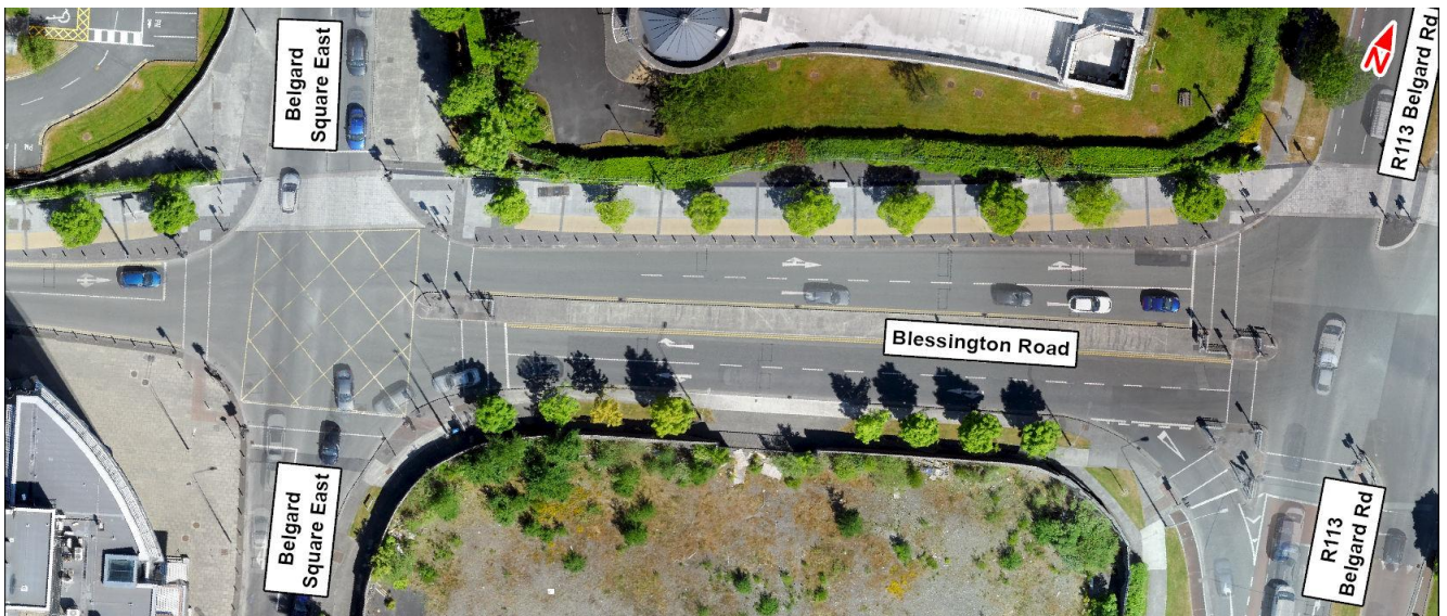
Image 5.7: Belgard Square East / Blessington Road Signalised Junction
